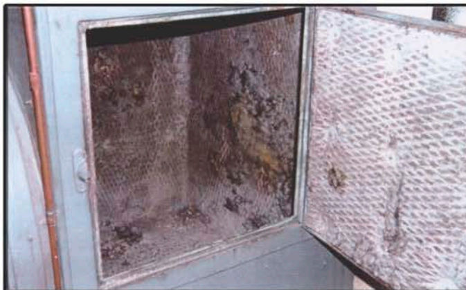
Mold growth and fiberglass delamination
